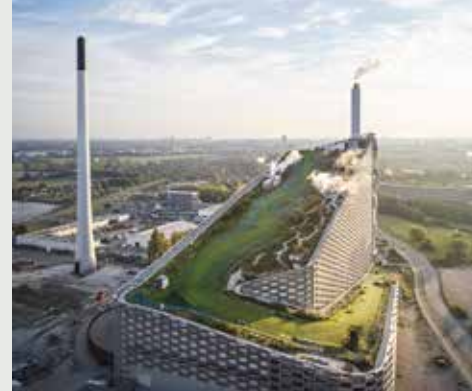
CopenHill / Amager Bakke
